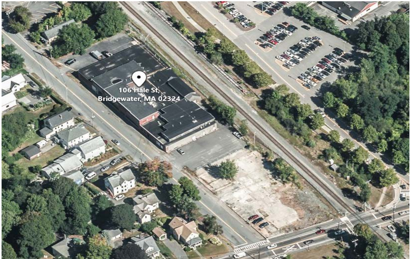
Aerial View looking down at 106 Hale Street site with former building still in place
