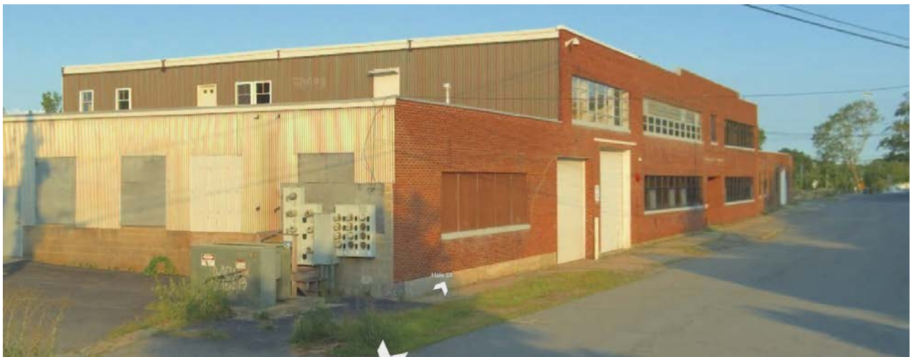
View of former building on 106 Hale Street property (since removed) looking south
