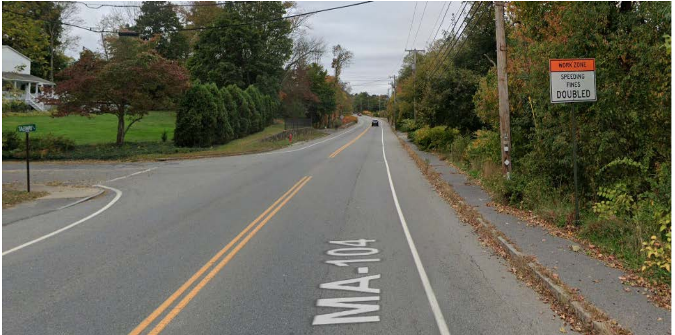
View of 1185 Pleasant Street looking west at intersection with Tabway Lane
