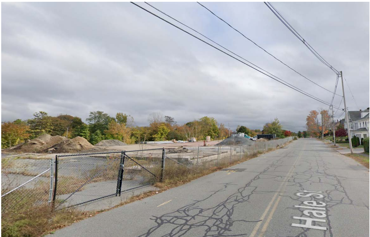
View of 106 Hale Street looking south
