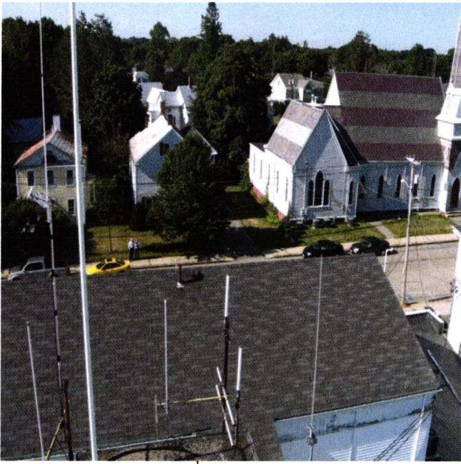
Shingle roof above 2 nd floor living quarters.
