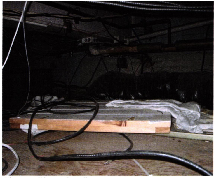
Above ceiling – first floor.
