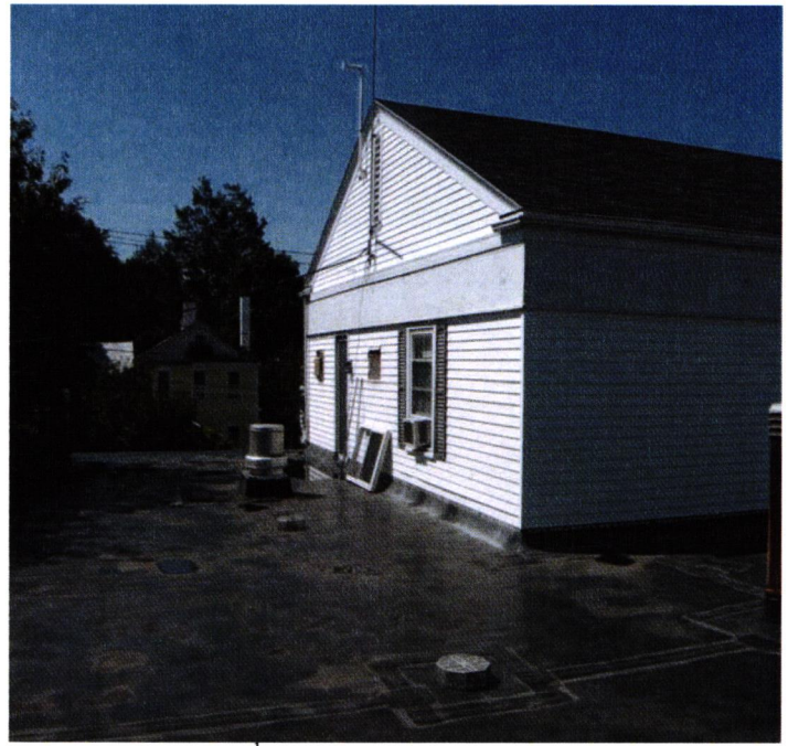
EPDM roof at 2 nd floor emergency exit.
