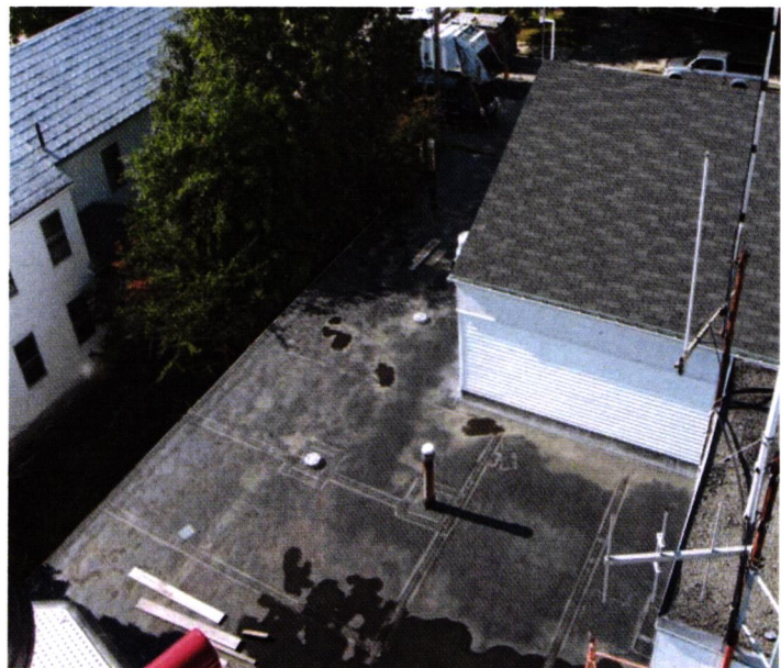
Membrane roof over 3-bay garage.
