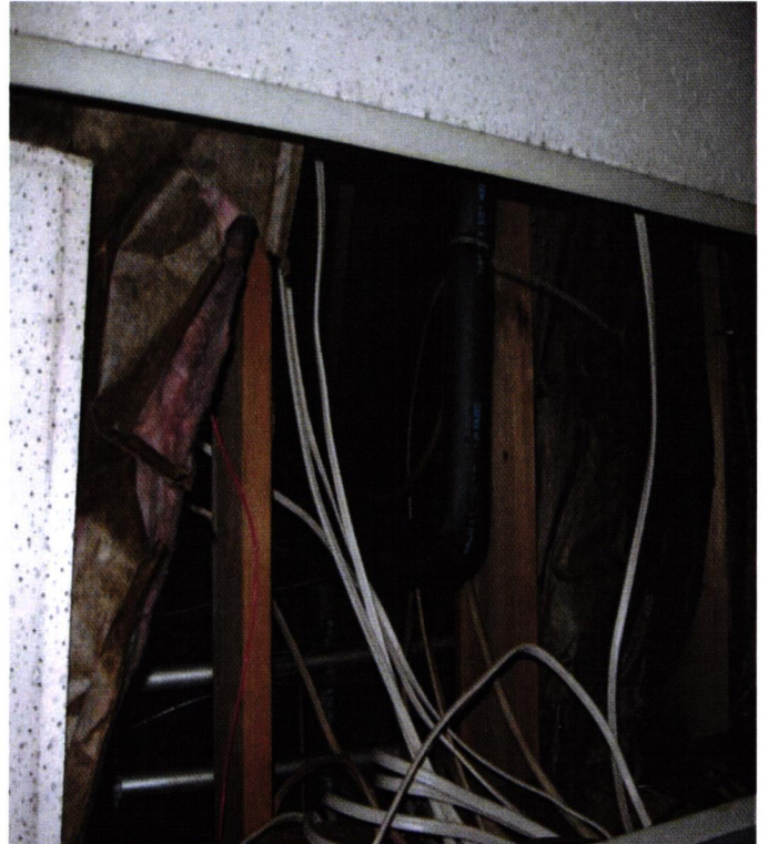
Above office ceilings.
