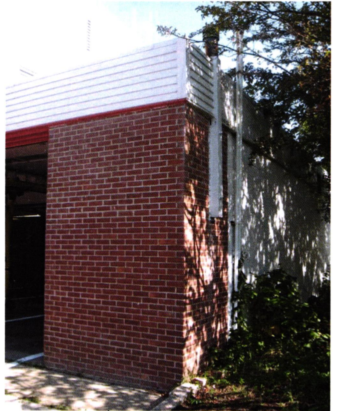
Brickwork at 3 rd bay door.
