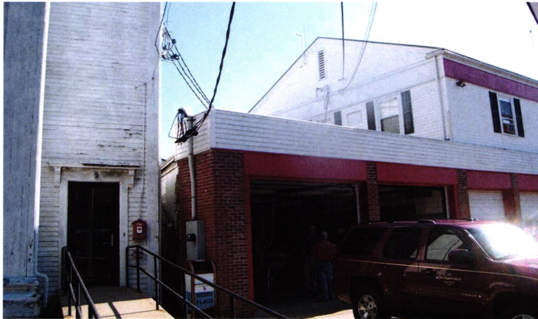
Photo 3.: Far left end of the front of the present station. Just about everything visible, except for the two brick piers at far right (above the vehicle's windshield) is not part of the original building.
