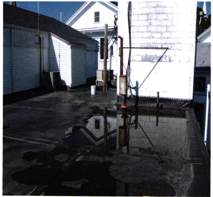
EPDM at base of tower.
