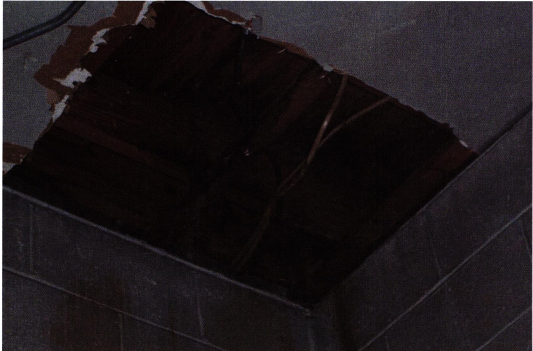
Photo 10.: Underside of roof framing at ceiling of Emergency generator Room.
