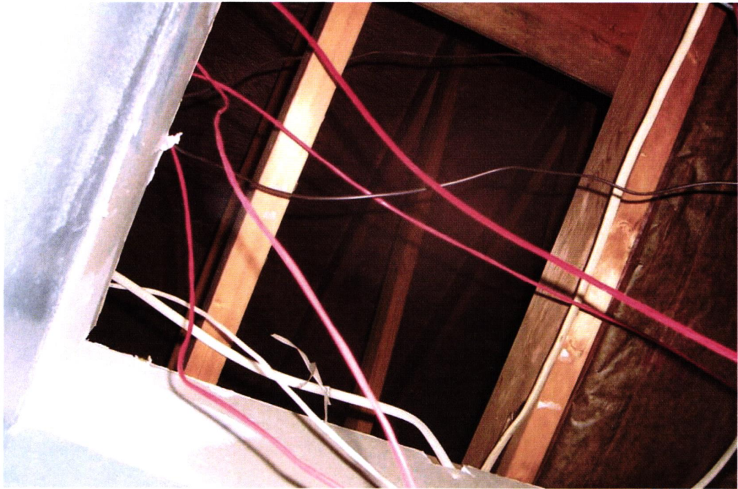
Photo 8.: View above ceiling of Second Floor, showing gable-pitched wood roof truss.
