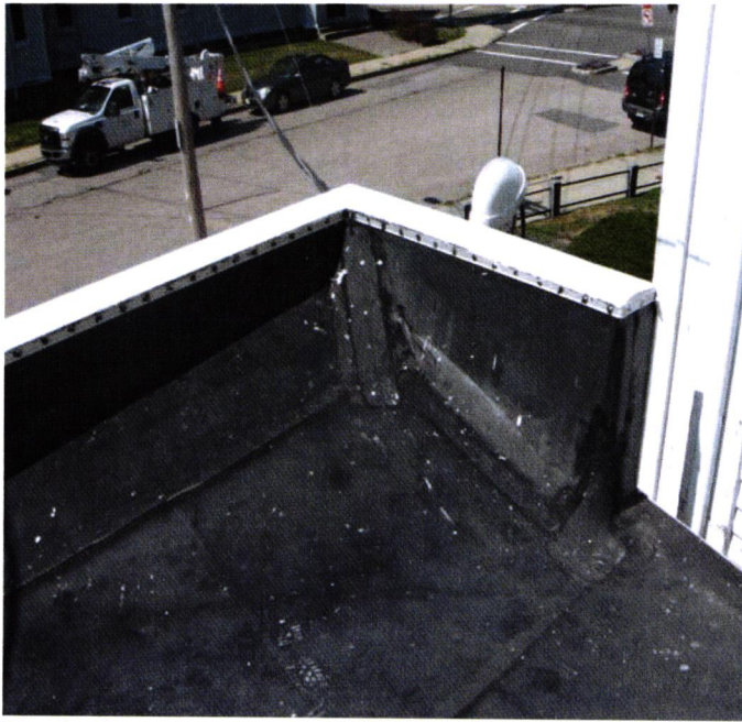
Typical curb flashing detail.
