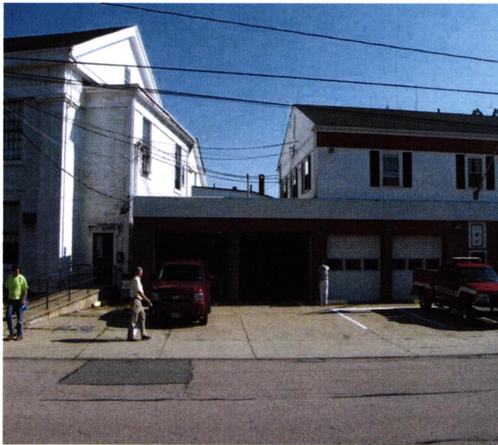
Front low ceiling bays.
